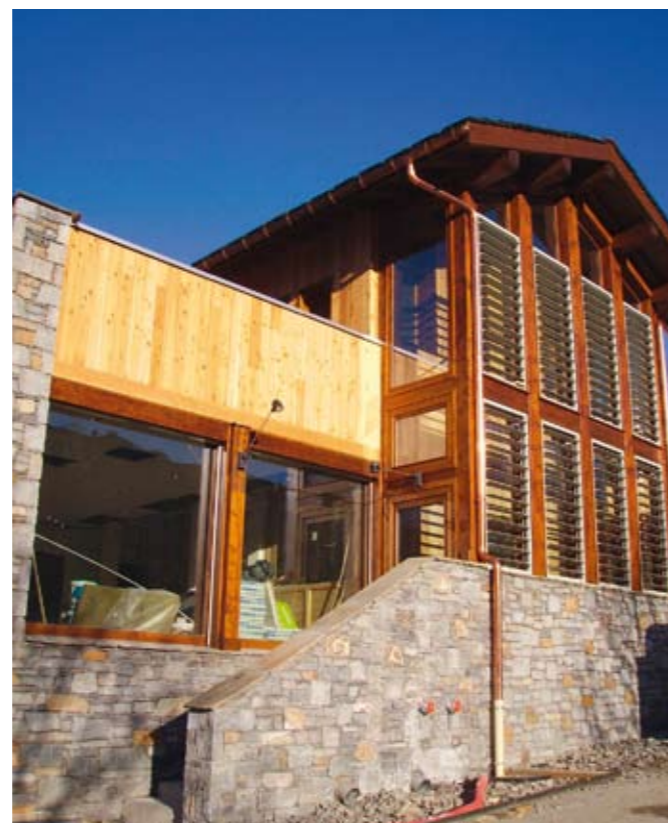
Strikingly aesthetic: the day nursery centre in Saint Martin de Belleville uses a minimum of heating energy.
